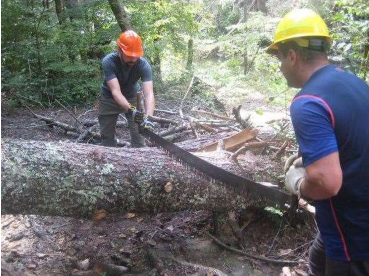
And MORE cross-cut work!
